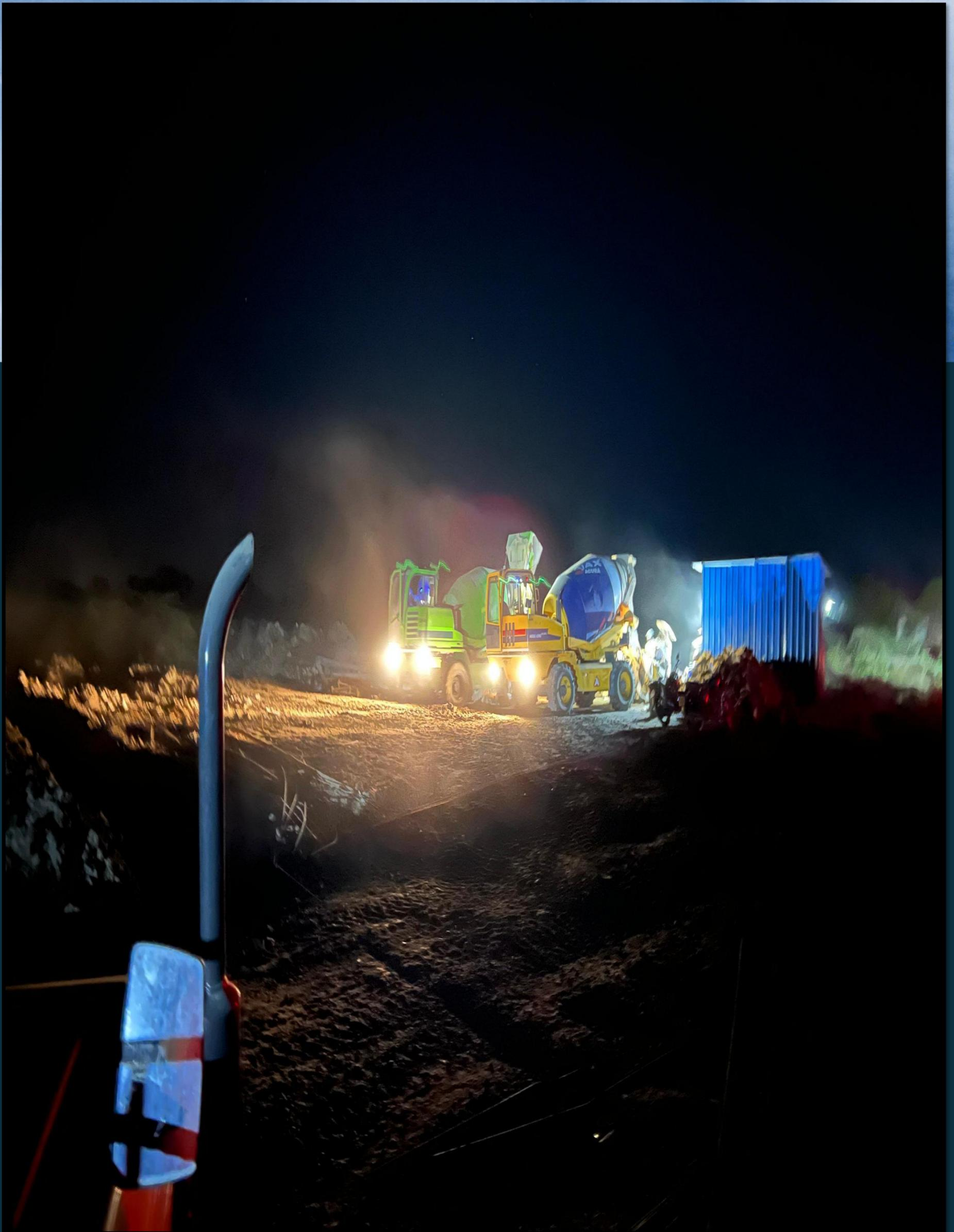
8. New Self Loading Mixers of Ajax & Swing Stetter of 4.5 & 4 Cubic Meter
